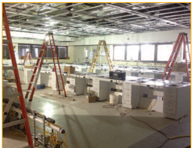
Workstations looking south, July 26, 2013
